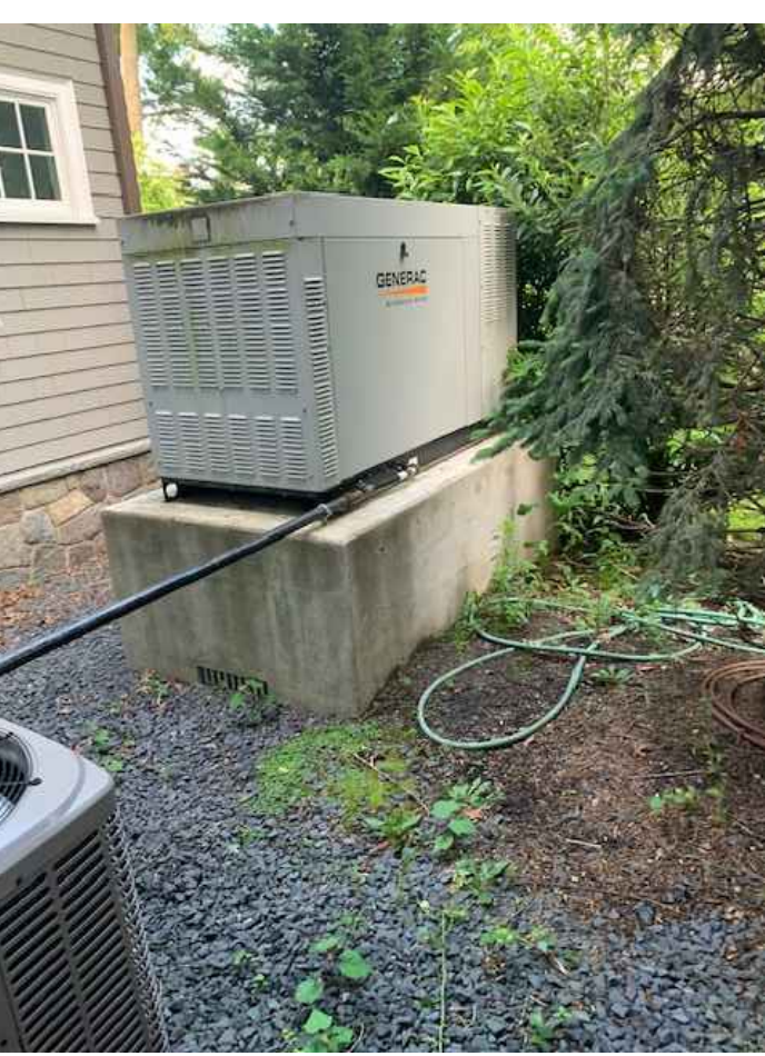
6) EXISTING AC UNITS AND GENERATOR LOCATED ADJACENT TO GARAGE AT EAST SIDE OF HOUSE. PROPOSED POOL EQUIPMENT TO BE SITED ADJACENT TO EXISTING MECHANICAL UNITS. POOL EQUIPMENT WILL BE SET ON A RAISED CONCRETE PAD TO BE SET AT MINIMUM ELEVATION +/- 13.0 OR SLIGHTLY ABOVE FLOOD ELEVATION
