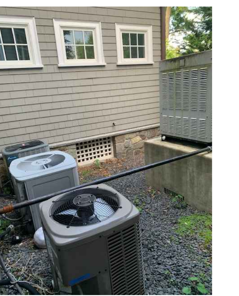
6) EXISTING AC UNITS AND GENERATOR LOCATED ADJACENT TO GARAGE AT EAST SIDE OF HOUSE. PROPOSED POOL EQUIPMENT TO BE SITED ADJACENT TO EXISTING MECHANICAL UNITS. POOL EQUIPMENT WILL BE SET ON A RAISED CONCRETE PAD TO BE SET AT MINIMUM ELEVATION +/- 13.0 OR SLIGHTLY ABOVE FLOOD ELEVATION
