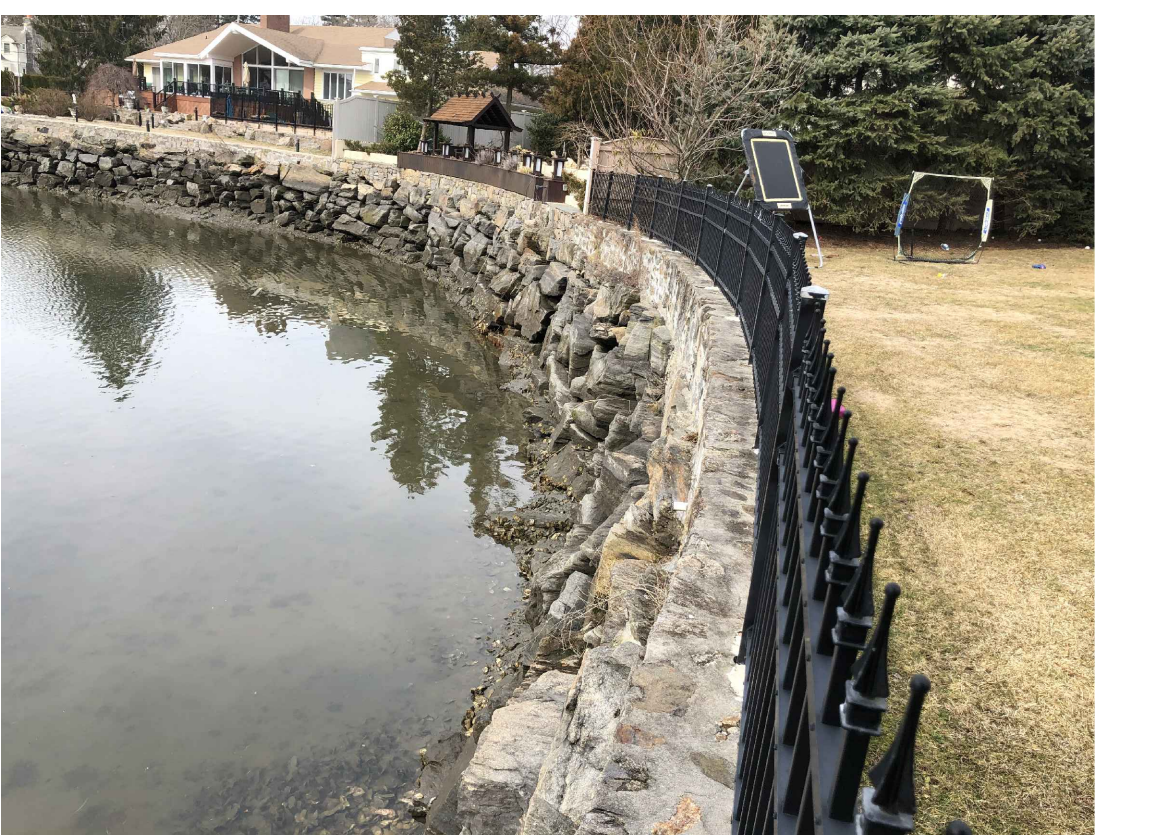
2 REAR OF PROPERTY BACKS UP TO SPANISH COVE. EXISTING ALUMINUM FENCE TO SERVE AS POOL SAFETY FENCE W/ MODIFICATIONS AS REQUIRED TO MEET NEW YORK STATE POOL CODE.
