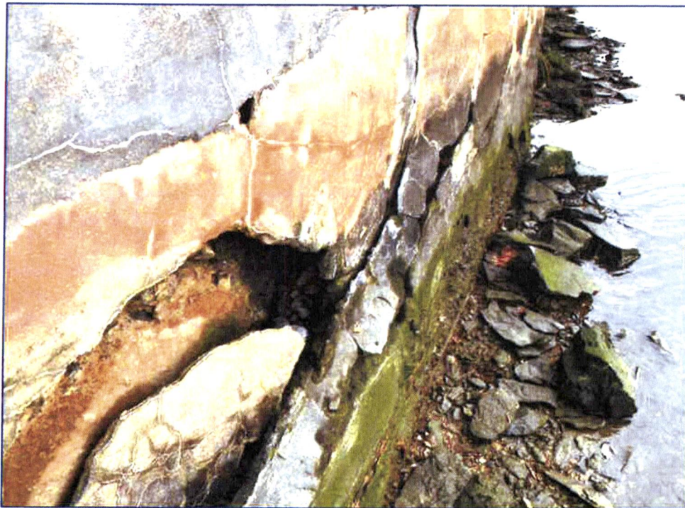
Photograph 6 – Existing Deteriorated Stone & Concrete Wall (Image Dated 12-5-2018)
