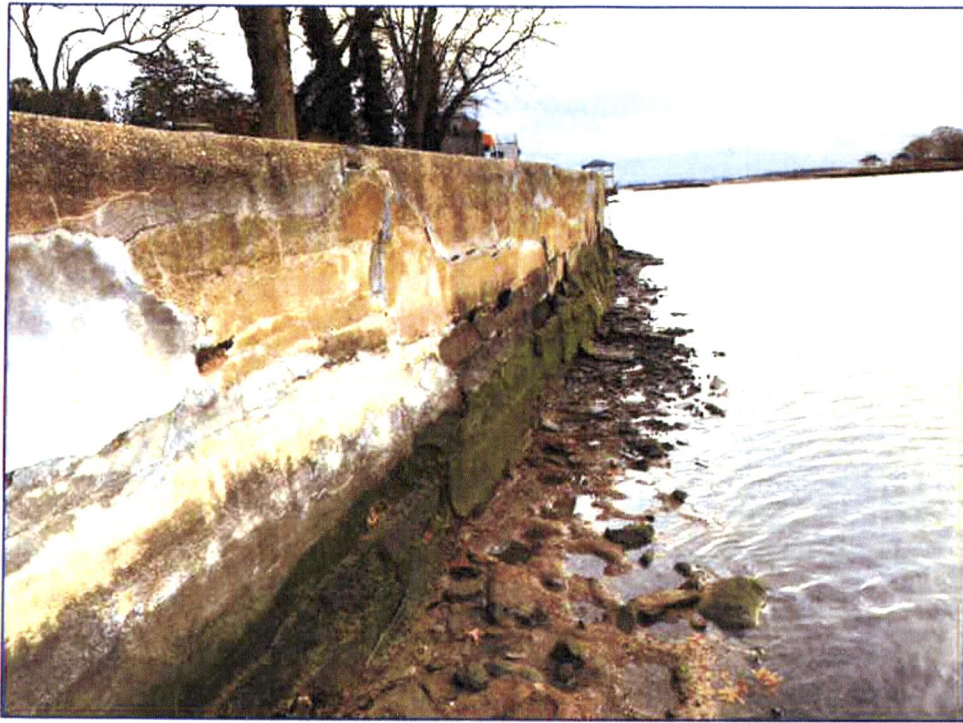
Photograph 5 – Existing Deteriorated Stone & Concrete Wall (Image Dated 12-5-2018)
