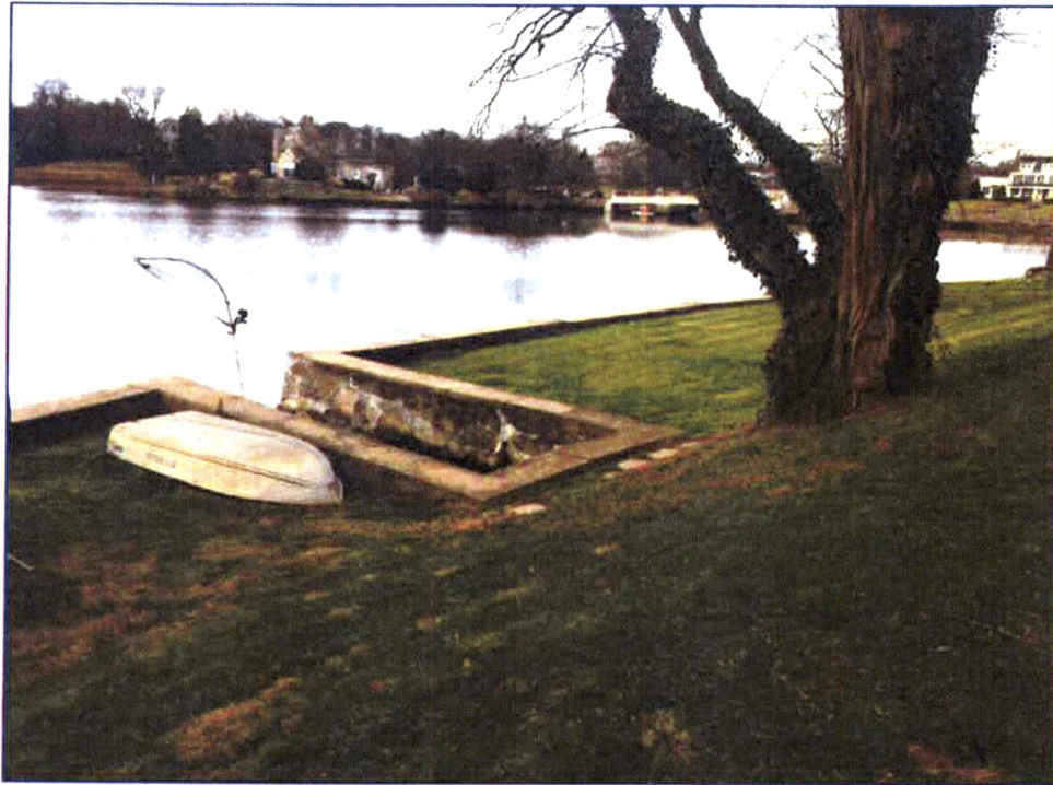
Photograph 1 – Existing Deteriorated Stone & Concrete Wall. (Image Dated 12-5-2018)
