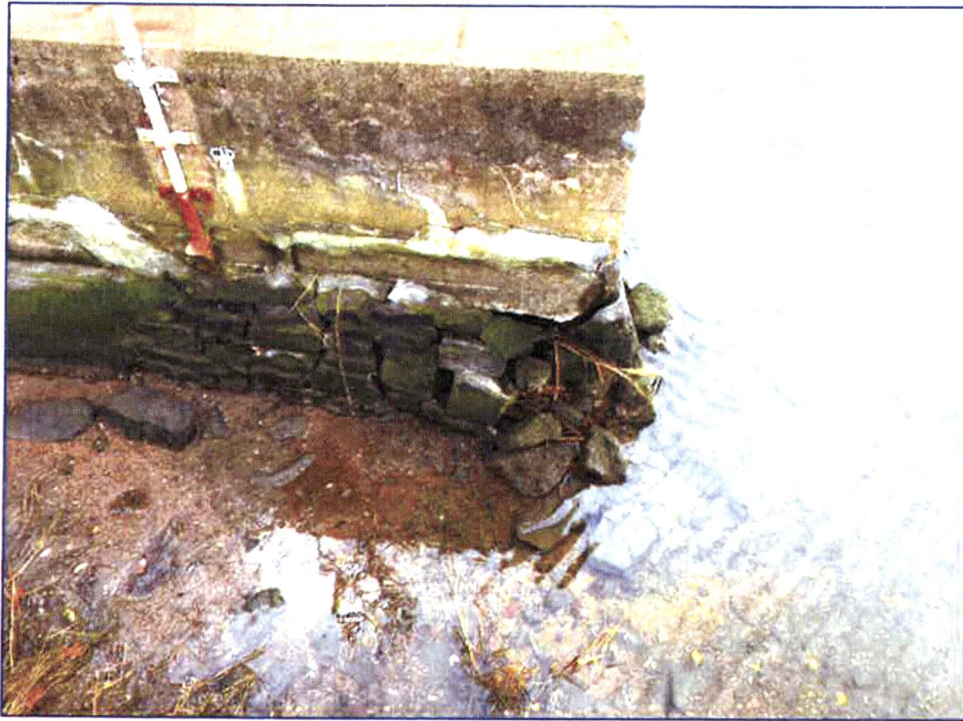
Photograph 3 – Existing Deteriorated Stone & Concrete Wall (Image Dated 12-5-2018)
