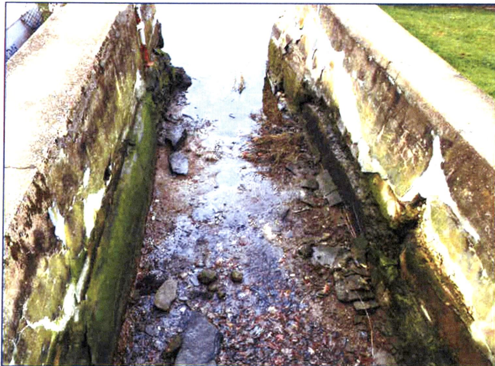
Photograph 2 – Existing Deteriorated Stone & Concrete Wall. (Image Dated 12-5-2018)
